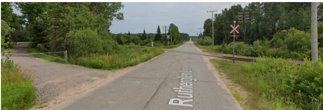
Photo Nine: Existing Signalized Crossing at Rutherglen Line facing South
