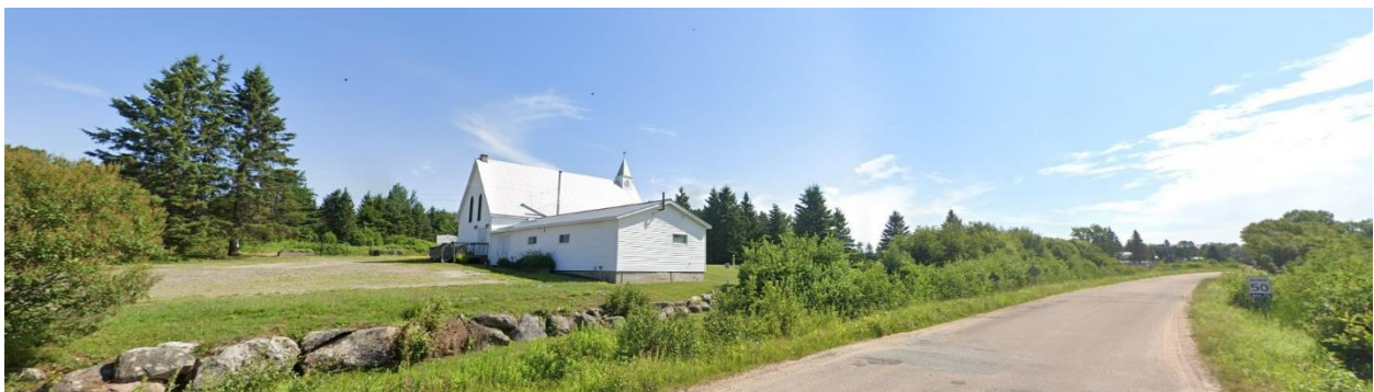
Photo Three: Facing East along Trunk Road South of St Margaret's Anglican Church
